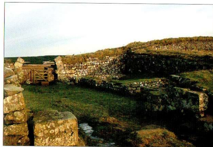
The base of the arched gateway survives at Milecastle 37
